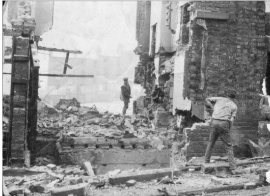
On the demolition - Bruce in the fore ground - 1965
