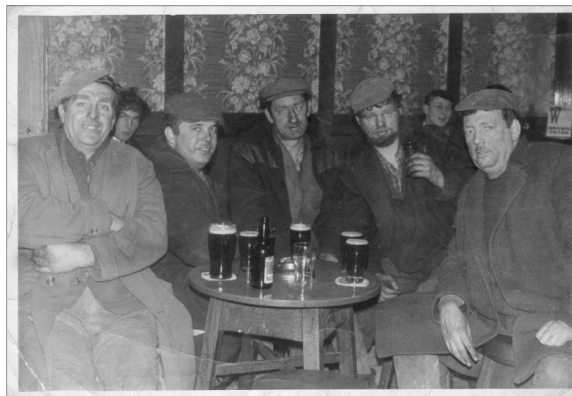
Demolition team - Bruce 4th from the left - in the Caledonian pub, Lime Street, before they knocked it down! - 1966
